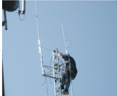
Danny Britton KB4TEP working off top of the KE4RX Tower
